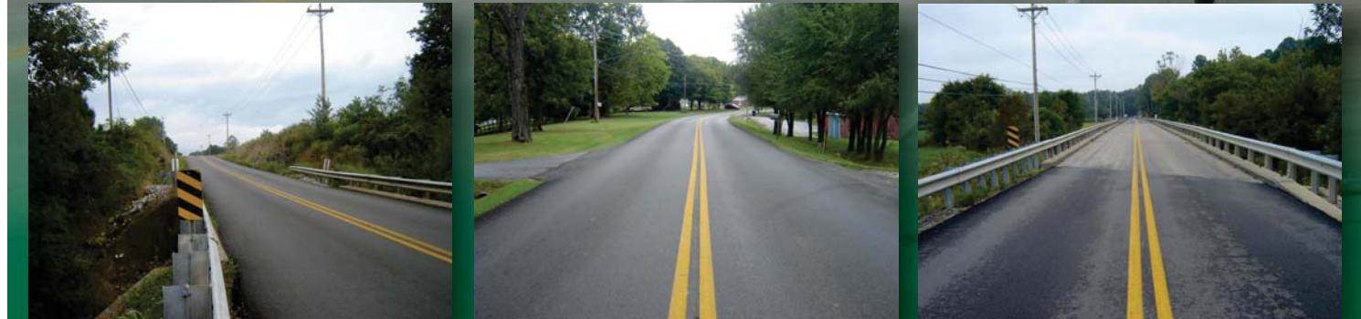
Black Rock Creek Bridge
